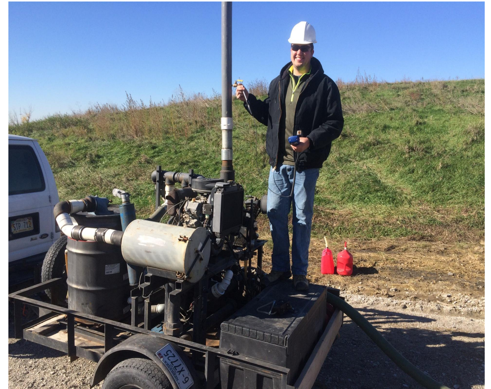
Taking exhaust readings during a pilot study for the installation of a methane mitigation system at the Cedar Island Landfill in Bellevue, Nebraska.
